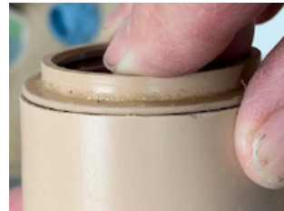
Fig 14. You should not see the O-ring when fully seated and glued in place.
