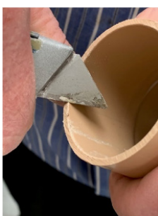
Fig 12. Deburr the edges and sand to smooth the cut end. Use caution with debris.
